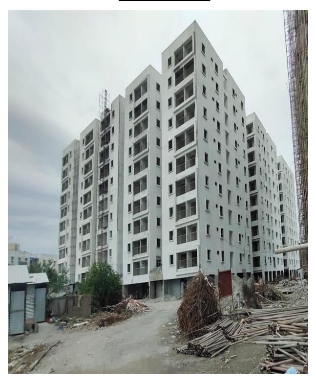
**Block D1:** External plastering overall 95% completed. 1st Coat Primer 95% completed.
