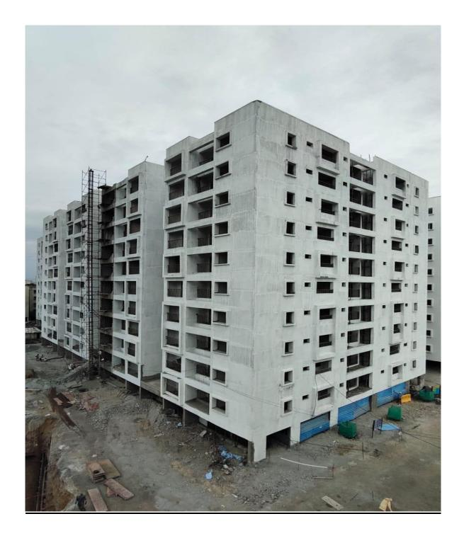
**Block D2:** Over Head Water Tank 100% completed. Lift installation works on progress. Terrace weathering course on progress. External Painting works on progress
